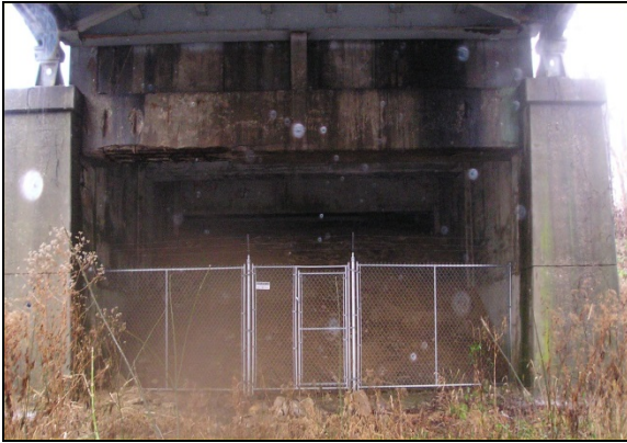
Photo 12 and 13: Bridge Design Mimicking “Cave-like” Atmosphere
